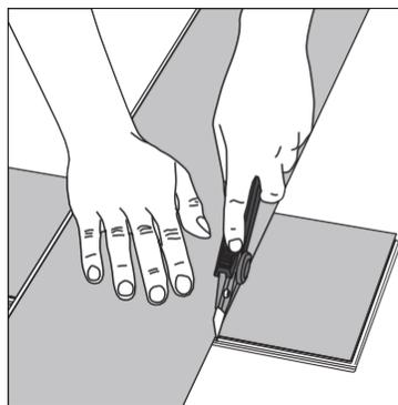
④ To cut the plank, use a simple utility knife and ruler, and with the top side facing up, cut heavily and several times on the same axis. The knife will not go through the surface but make a deep cut. You can then lift one half of the plank using your other hand to hold down the second placing it very close to the cut. The plank will split naturally.
